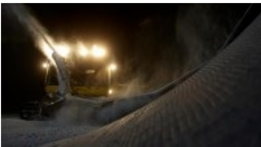
Gateway Parks Freestyle Park Build at Night
